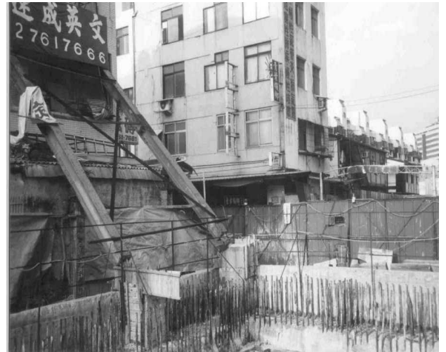
Figure 4. Underpinning at JDB- Exit A site
