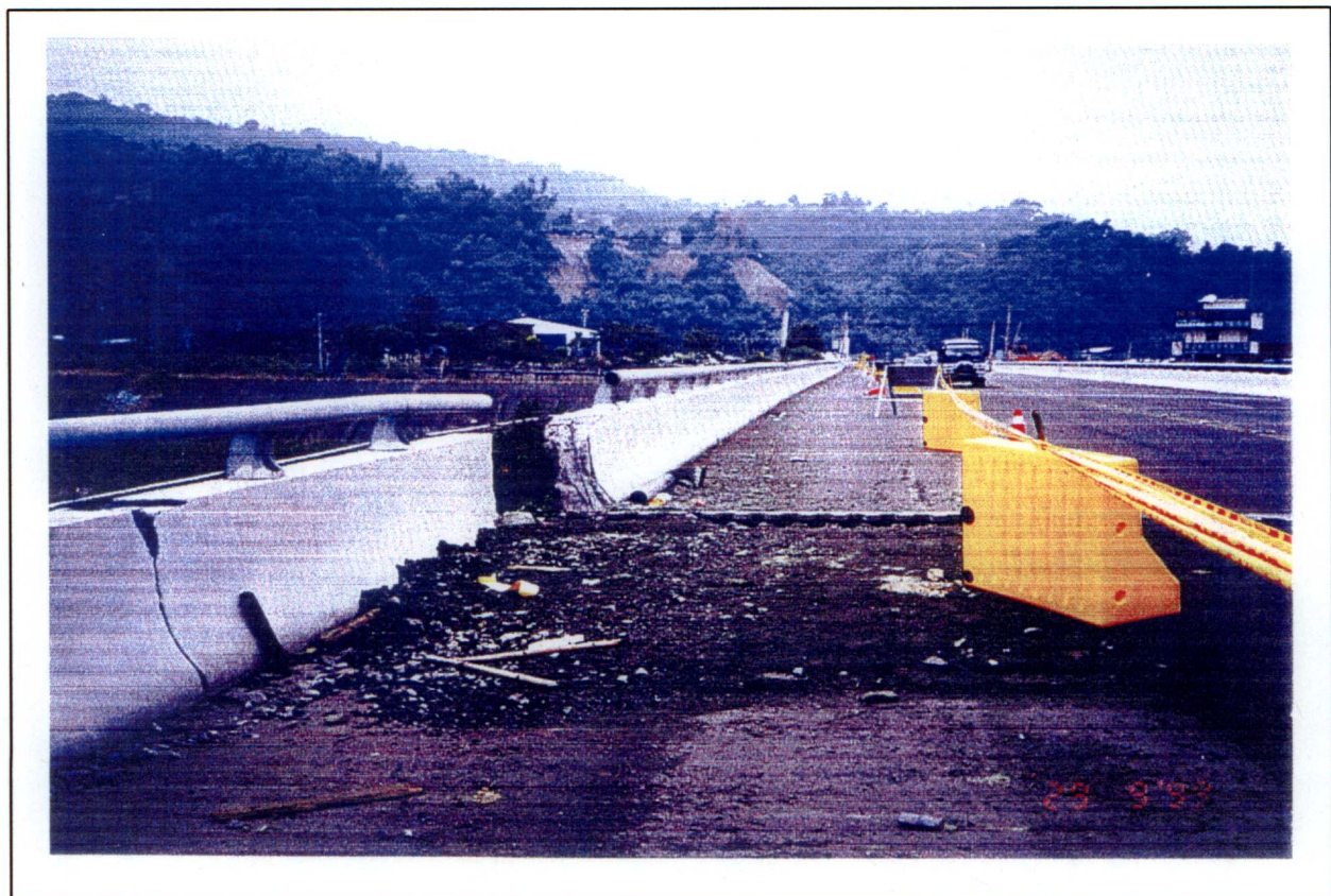
Fig 3: Conditions of Slab Displacement and Opening to Traffic
