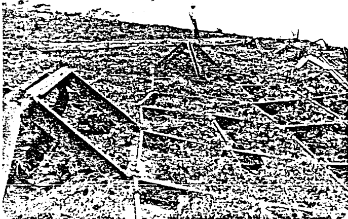
Fig. 11 Photo Showing Cone shaped Concrete Grids
