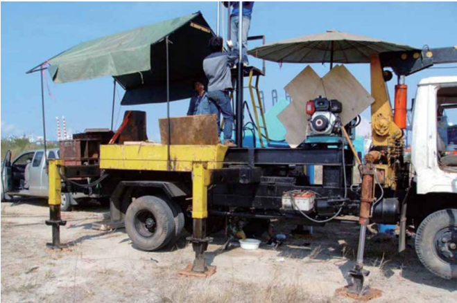
Nong Saeng Natural Gas Power Project, Thailand
