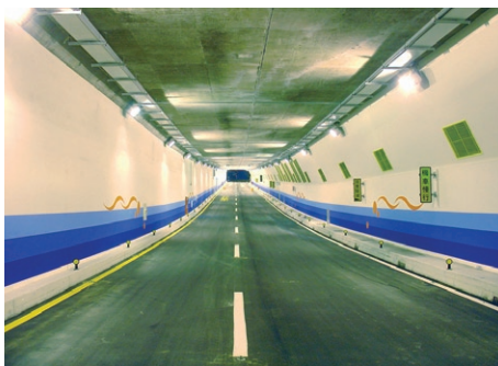
Fushing North Road Underpass
