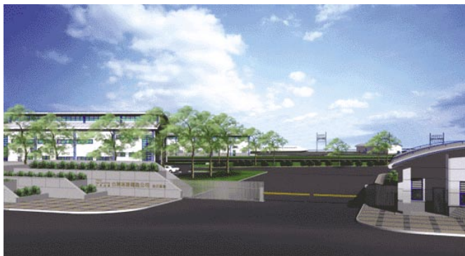
High Speed Rail Wujih Depot
