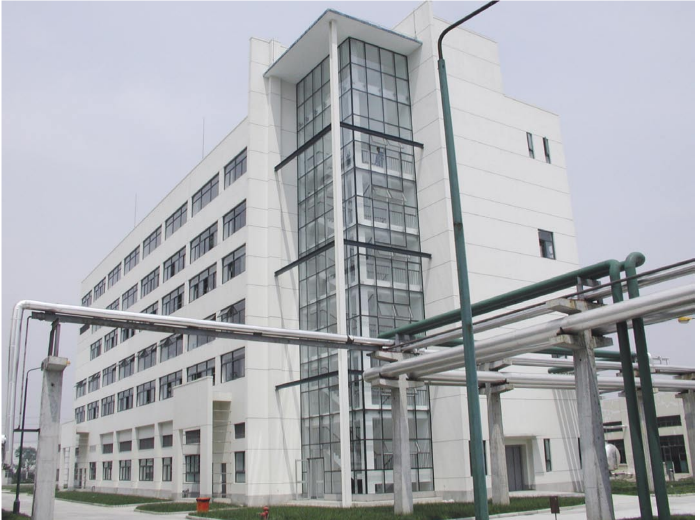
The GMP Transformation Shop of Hutchison Pharmaceutical (Shanghai)
